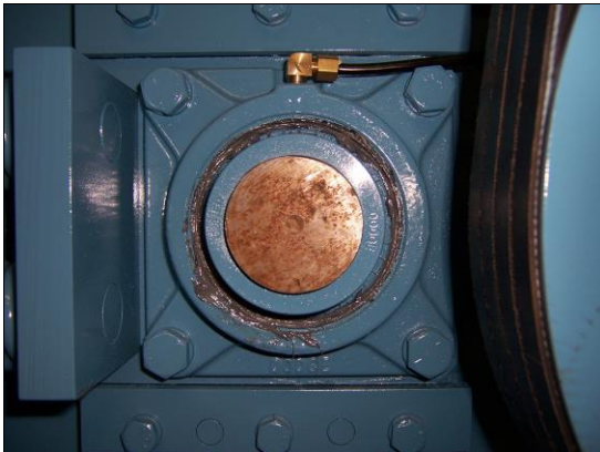
Figure 1. A correctly greased bearing has grease purging around the perimeter.
